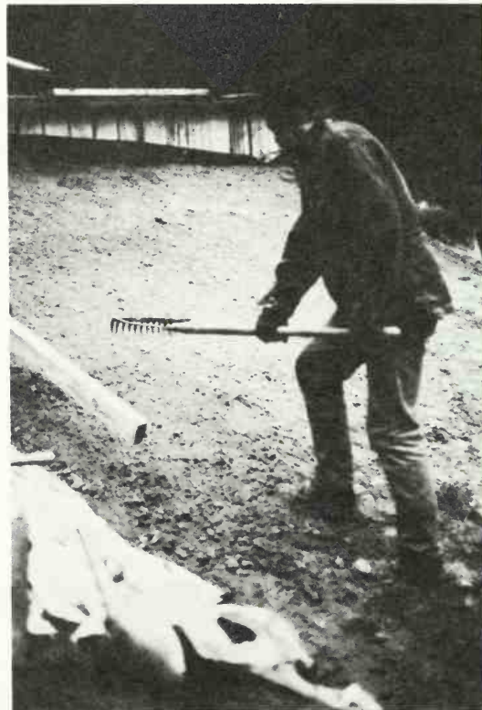
Incorrect procedure for raking first layer of earth smooth is demonstrated here. Tines of rake should not be used, but backside, so as not to risk tearing polyethylene.
